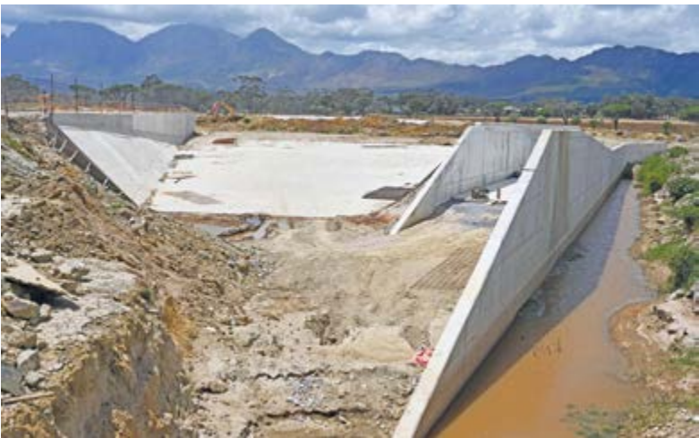
Concrete improvement: This transition structure is among the measures implemented at Sir Lowry's river to support river flow and help prevent future floods.
