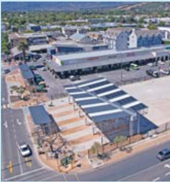
A PTI to be proud of: The new and improved Somerset West public transport interchange (PTI) on the corner of Andries Pretorius and Victoria streets is operational. Every weekday, the facility serves some 1 000 commuters, travelling to destinations such as Lwandle, Macassar, Firgrove, Strand, Nomzamo, Sir Lowry's Pass Village, Zola, Khayelitsha, Stellenbosch and Grabouw.
