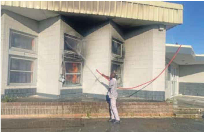
Bad end to the day: The Khayelitsha library building caught fire on 1 February, just as staff were locking up for the day. The cause has yet to be determined.
